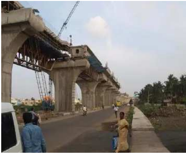
MRTS Phase II extension project in progress
