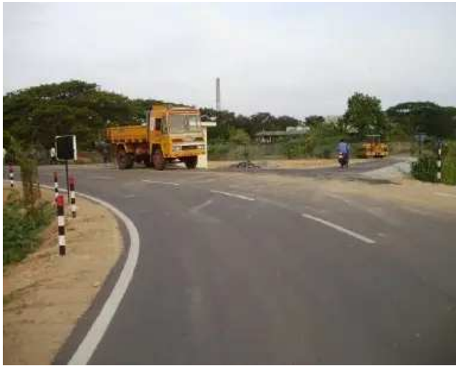
Widening and Strengthening of Ariyalur - Vilangadupakkam road under TNUDP III
