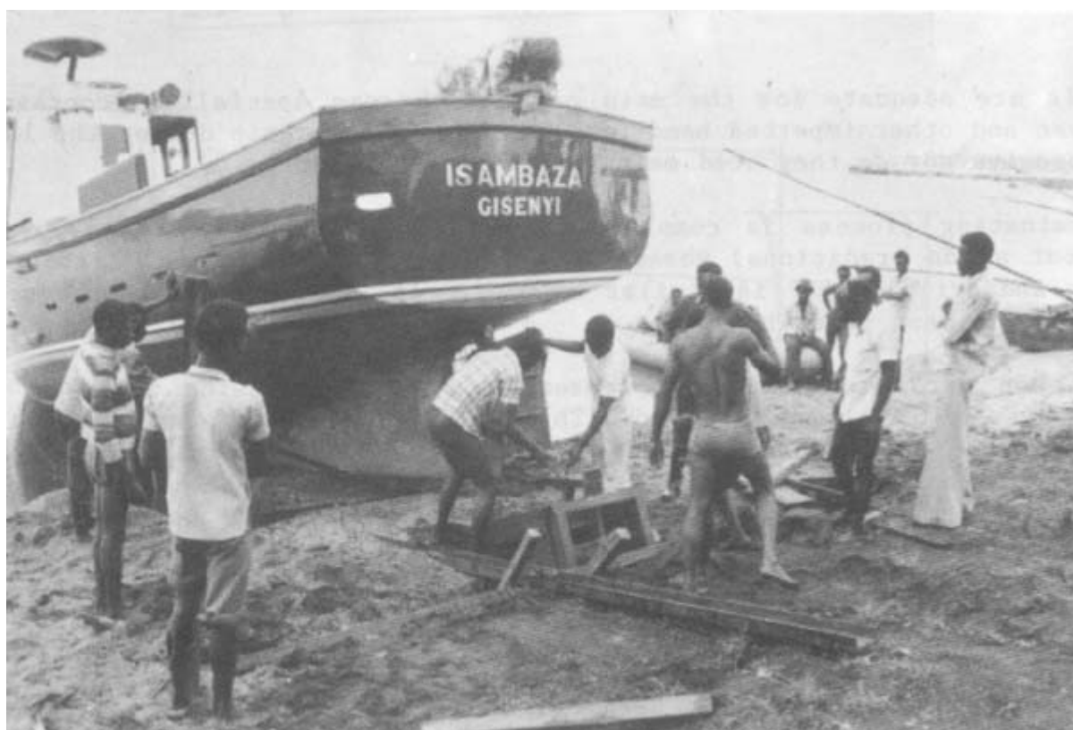
Figure 38 Hauling out a fishing vessel
