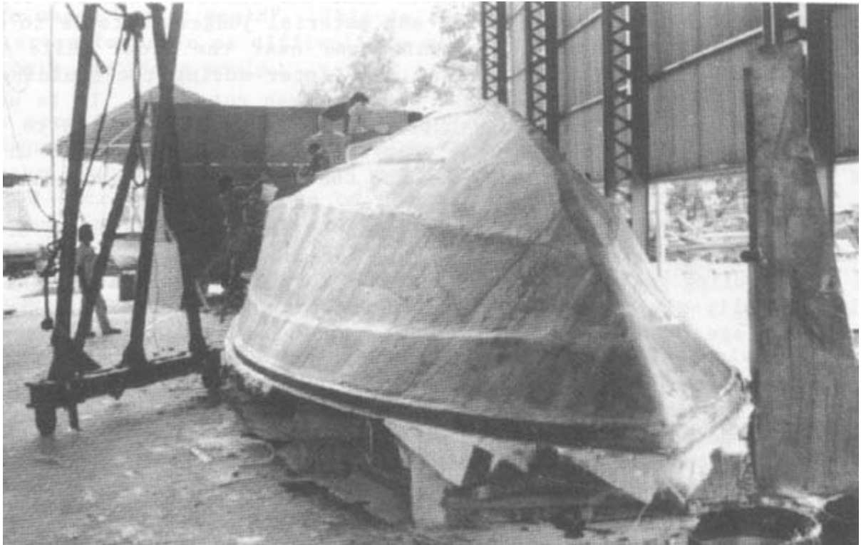
Figure 26 Mould construction
