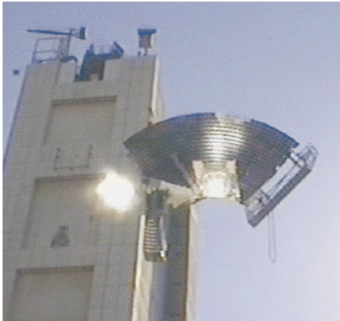
Fig. 2-22 Reflector in the Weizmann's Institute solar power tower /SolarPaces 2001/
