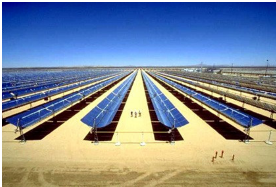
Fig. 2-12 SEGS plant in Kramer Junction, California /SOLEL 2005/
