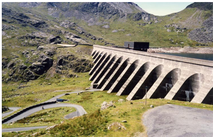
The Llyn Stwlan upper reservoir and dam of the Ffestiniog Pumped Storage Scheme in north Wales. The lower power station has four water turbines which can generate 360 MW of electricity within 60 seconds, an example of artificial energy storage and conversion.
