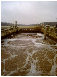
Using design knowledge to make better wastewater treatment facilities
