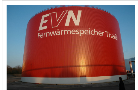
District heating accumulation tower from Theiß near Krems an der Donau in Lower Austria with a thermal capacity of 2 GWh
