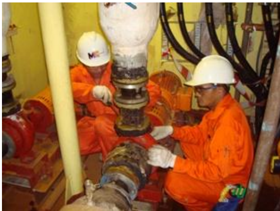
Chilled Water Pump Repairs FPSO Vincent Keppel Singapore
