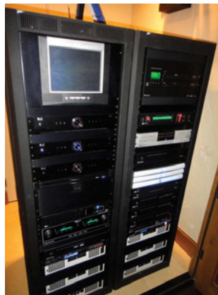
Universal Systems' Austin project incorporates Middle Atlantic Products' gangable WRK Series wide body equipment racks.
