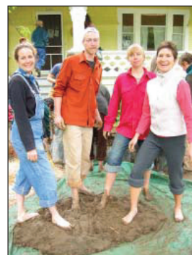
Mixing cob by foot
