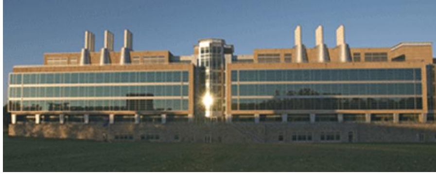
Figure 1.5 The new FBI laboratory in Quantico, Virginia.
