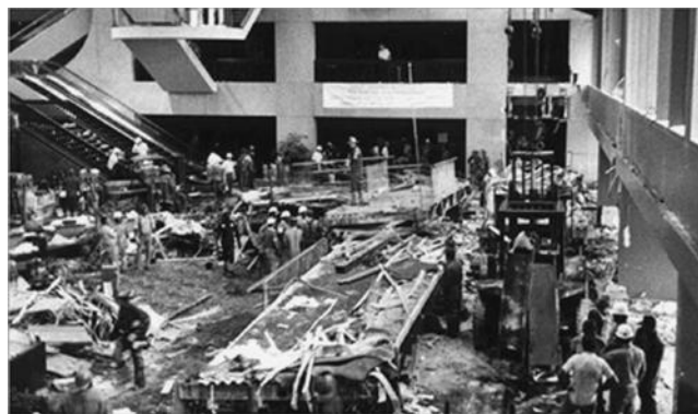
Figure 1.1 Wreckage of the collapsed Hyatt Regency Hotel in Kansas City. Associated Press file photo (with permission).
