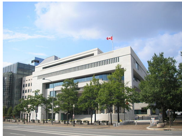
Canadian Embassy in Washington, D.C. showing planters being used as vehicle barriers, and barriers and gates along the vehicle entrance
