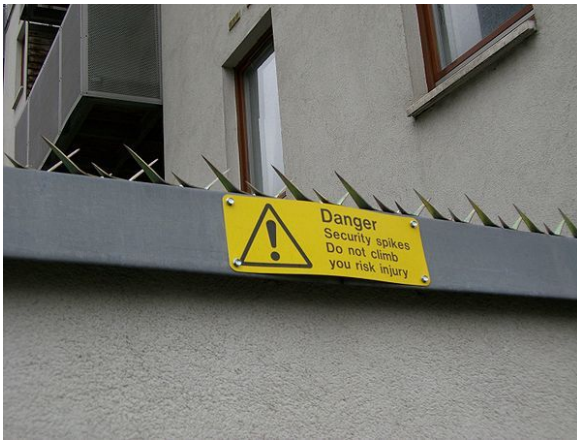
Spikes atop a barrier wall act as a deterrent to people trying to climb over the wall
