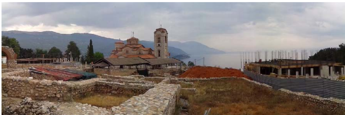
PHOTO 31: ARCHAEOLOGICAL STRUCTURES BETWEEN THE TWO DEVELOPMENTS WITH POTENTIAL TO BE AFFECTED BY WIND AND WATER EROSION
