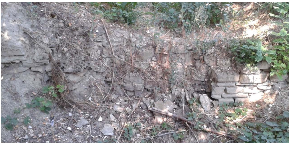
PHOTO 18: FLOOD AND RAIN EROSION OF STEEP ARCHAEOLOGICAL STRUCTURES ON LOWER TERRACE
