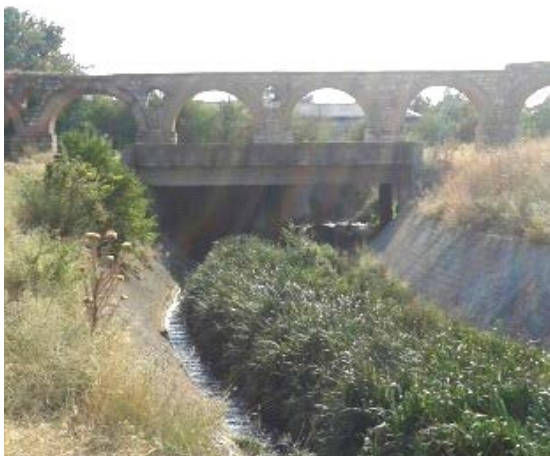
PHOTO 2: CANALIZED RIVER BED OF SEREVA RIVER UNDERNEATH PIERS 31-33 OF THE AQUEDUCT
