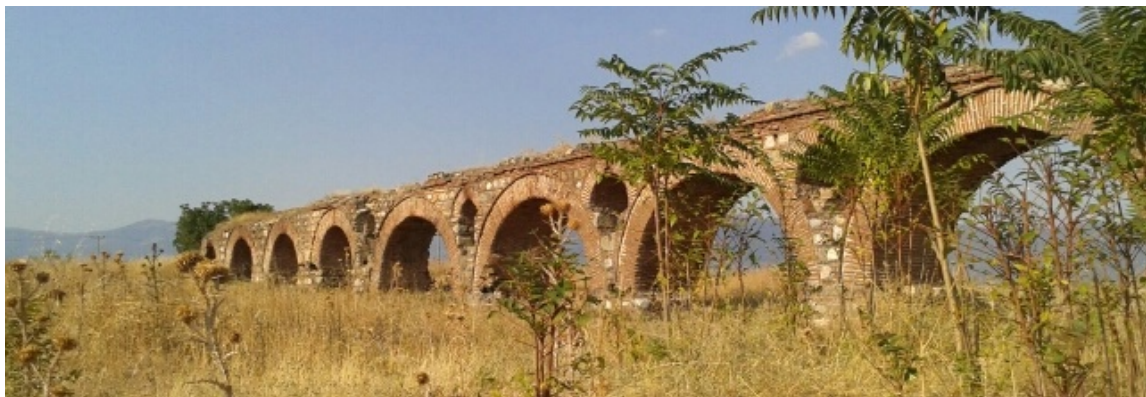
PHOTO 1: NORTHERN SECTION OF AQUEDUCT
