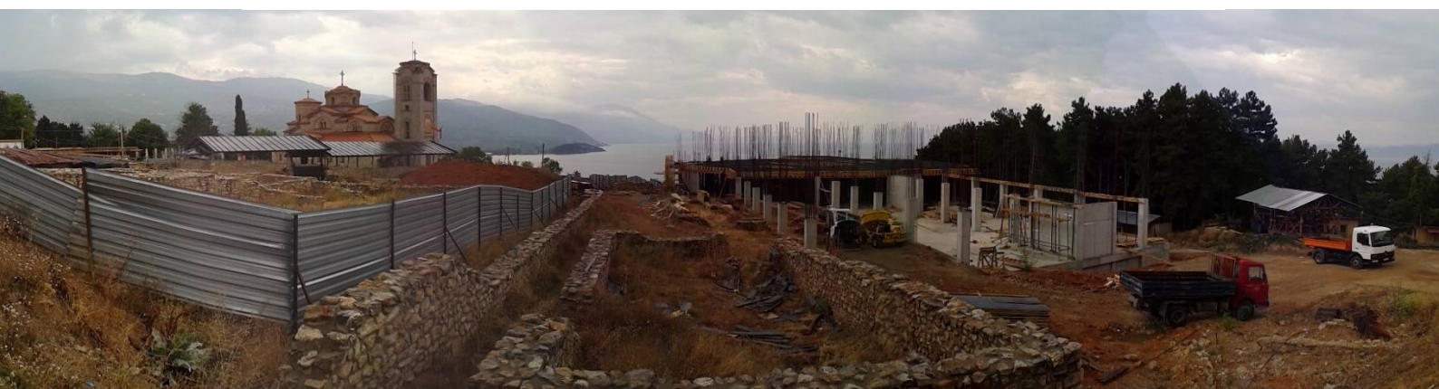
PHOTO 28: CONSTRUCTION OF THE ST. CLEMENTS UNIVERSITY COMPLEX WITH INTEGRATED MUSEUM ON THE WESTERN PART OF PLAOSNIK
