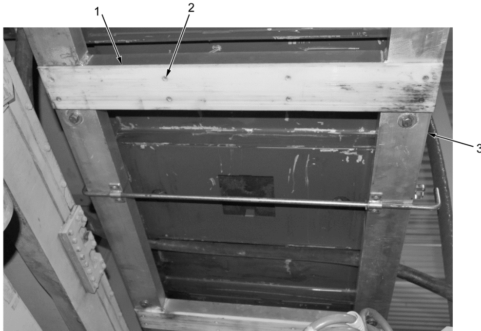
Figure 1. Generator Slide Pad Replacement.
