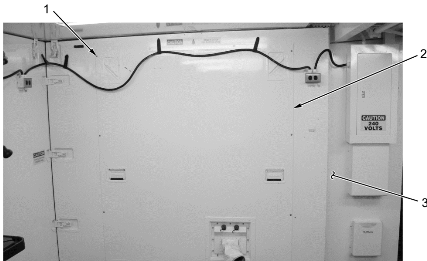
Figure 1. SEP Assembly Replacement.
