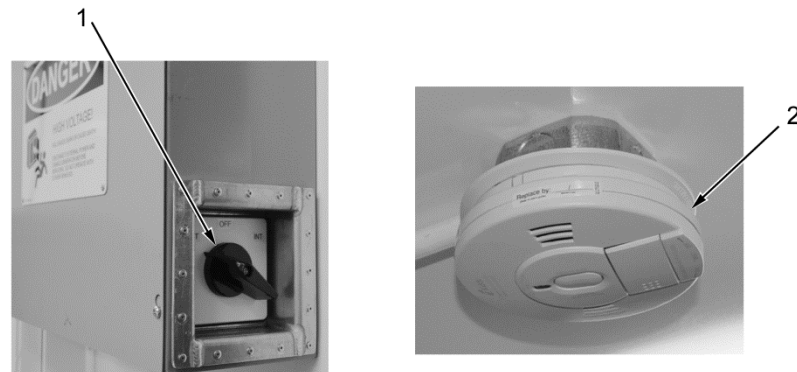
Figure 1. Selector Switch and Smoke Alarm.
