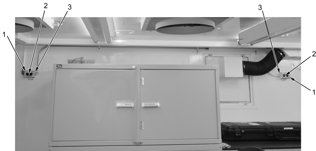
Figure 1. Outlet Covers Removal.
