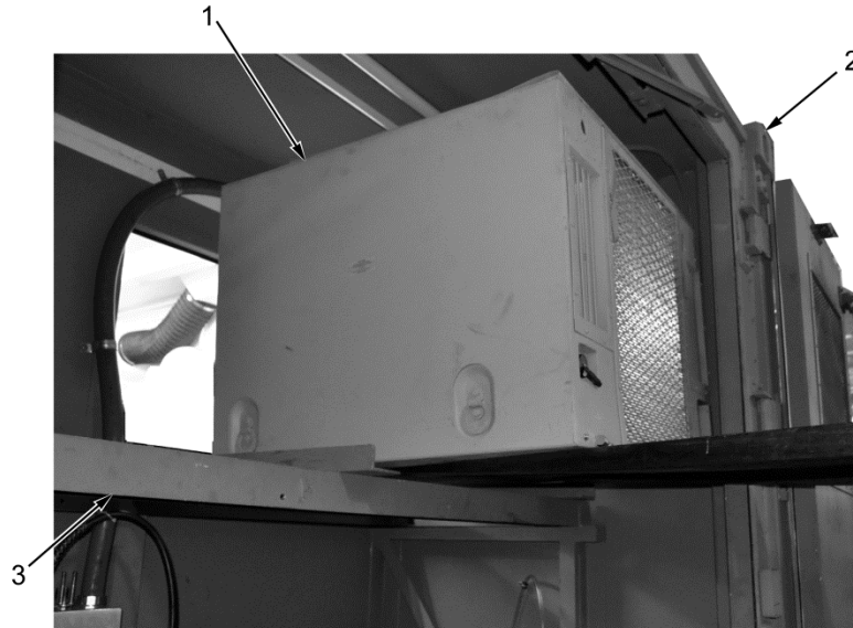
Figure 4. ECU Installation.
