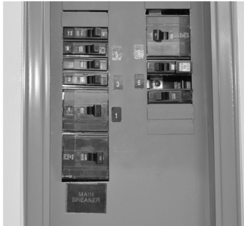
Figure 3. Circuit Breakers.
