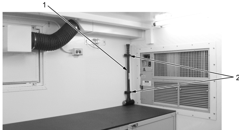
Figure 3. Sledge Hammer Installation.
