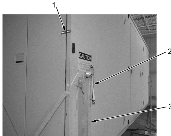
Figure 22. Aligning Sidewall and End Walls.
