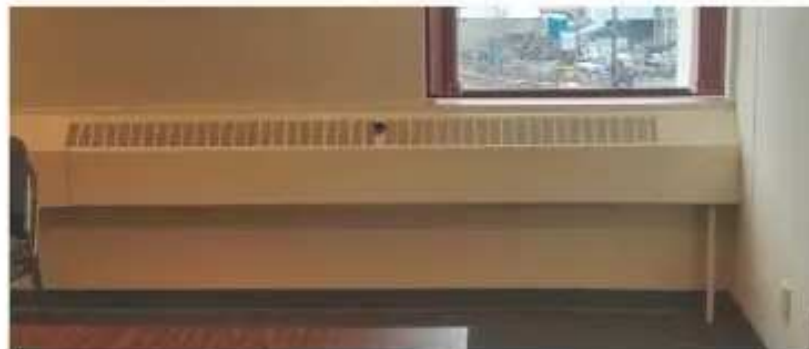
Figure 3 Perimeter Wallfin Radiators
