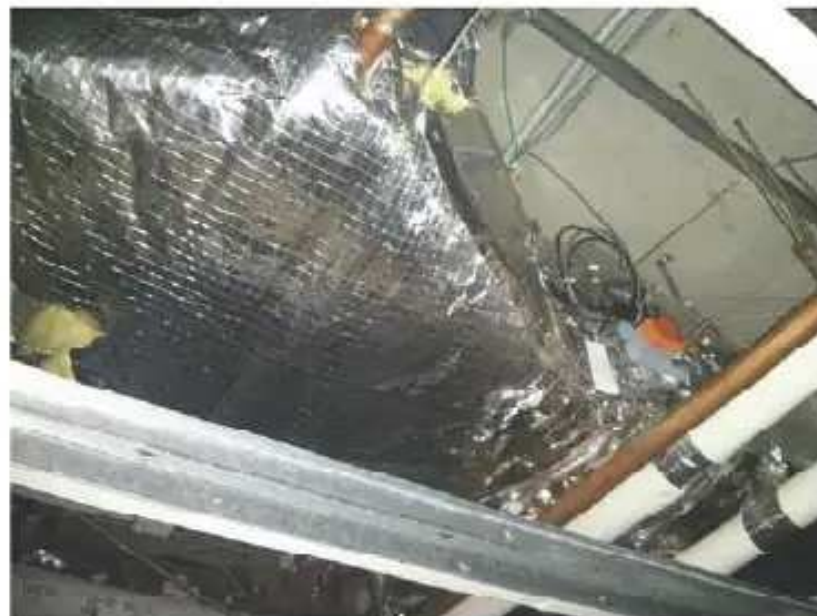
Figure 1 Zone Control Damper and Reheat Coil
