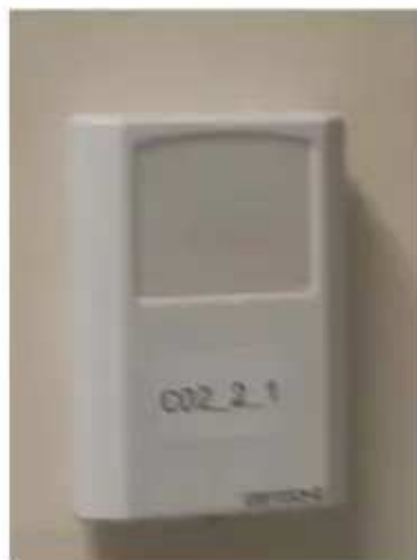
Figure 2 CO 2 Sensor for Demand Control Ventilation
