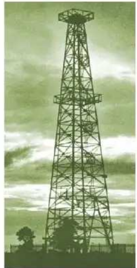
Fig. "Betch-still" used in Margherita Refinery Unit
