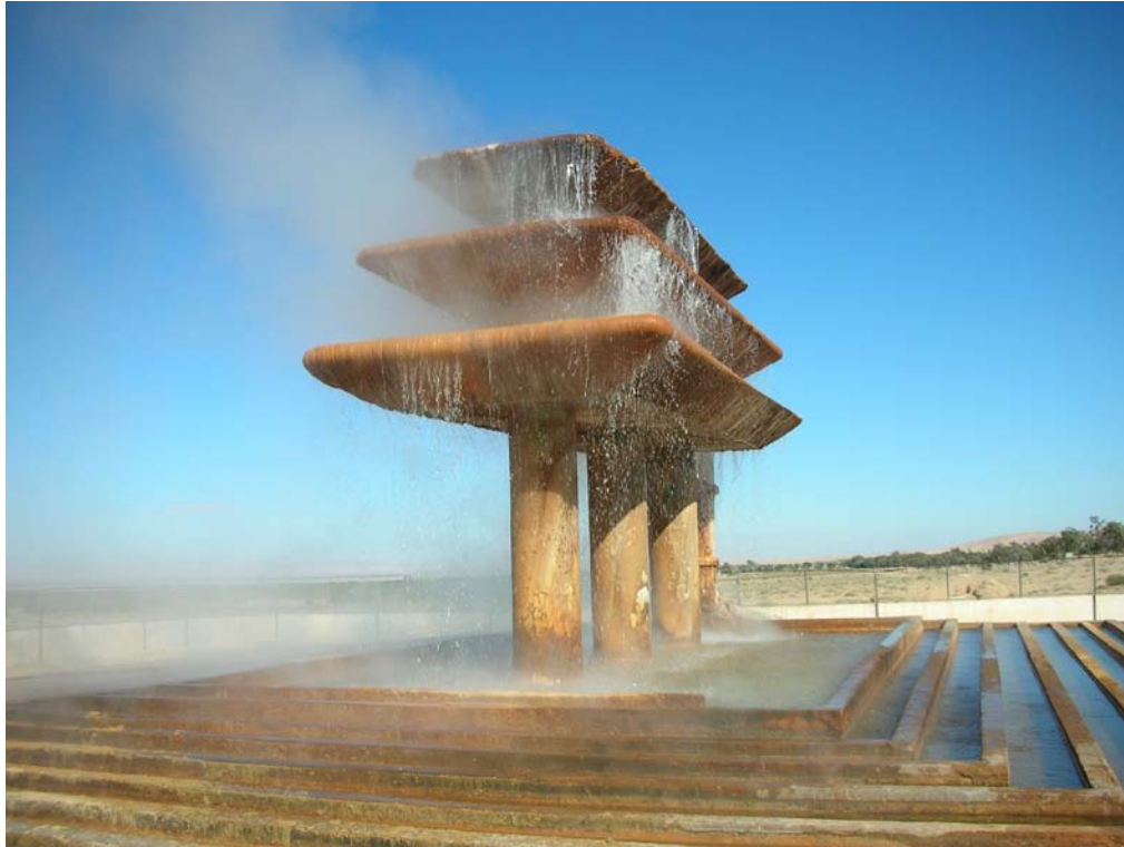
Figure 2: Cooling tower bringing geothermal water from the Sahara down to a temperature useable in irrigation
